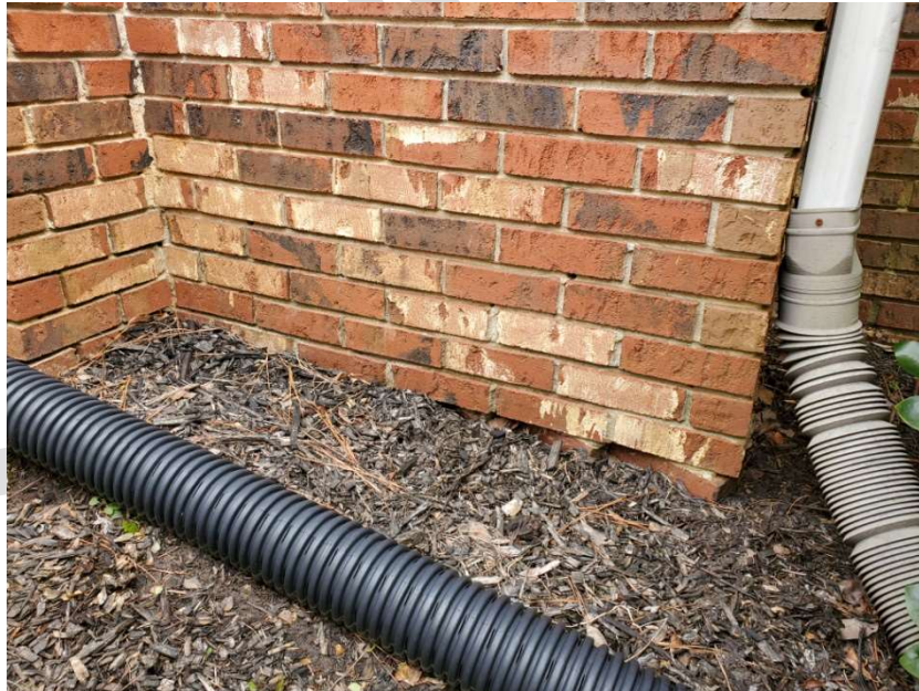
< Fig. 8 – Outside brick veneer at basement above >
