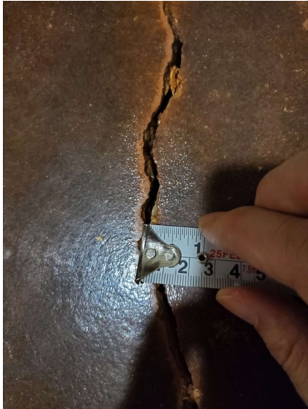
< Fig. 6 – Crack measure and slab settlement check >
