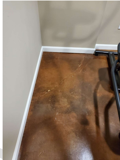
< Fig. 5 – Cracks on basement slab-on-ground >
